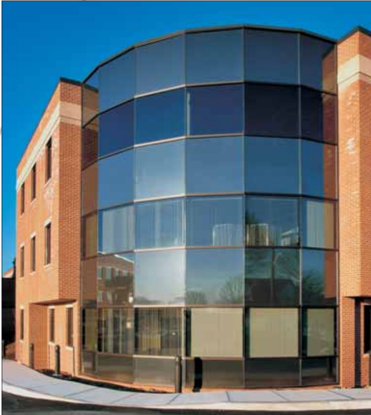
Addition to the 1948 Building at Ephrata Community Hospital for New Pharmacy and Medical Records Department
